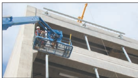
High in the sky, NAFCO crew members install structural steel to aid in the support of the fabric.
