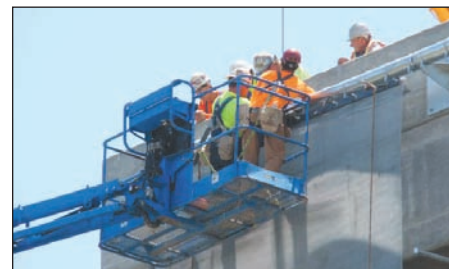
NAFCO workers install the first of the 3/8" x 9 ga. wire mesh panels.
