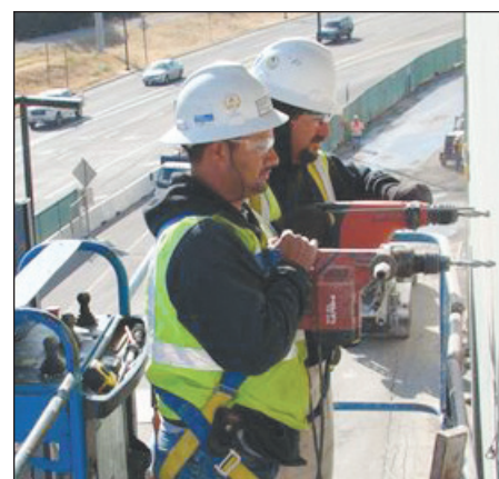
NAFCO crewmen Ricky Gonzalez and Oscar Amezcua drill holes for 3/4" x 7" S.S. Hilti anchors to mount the support plates for the 6-5/8" horizontal rails.
